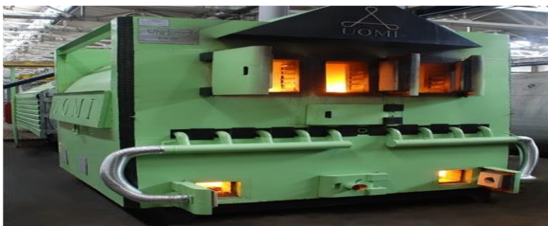
Fig.2 Incineration of solid waste
